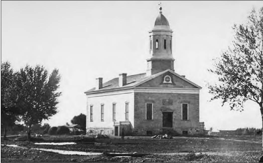
Figure 10. Finished Original Provo Tabernacle, photo taken prior to 1883 (Image courtesy of the Utah State Historical Society).
