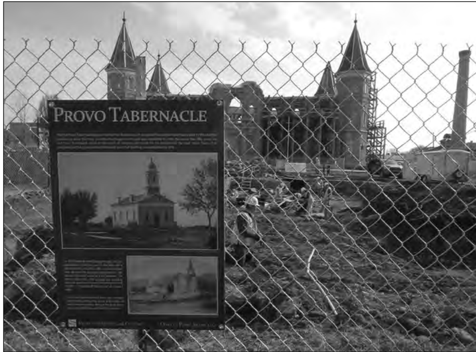
Figure 13. One of the interpretive signs produced by OPA and the MPC to provide visitors to the site with information about the project (Photo courtesy of Charmaine Thompson).
