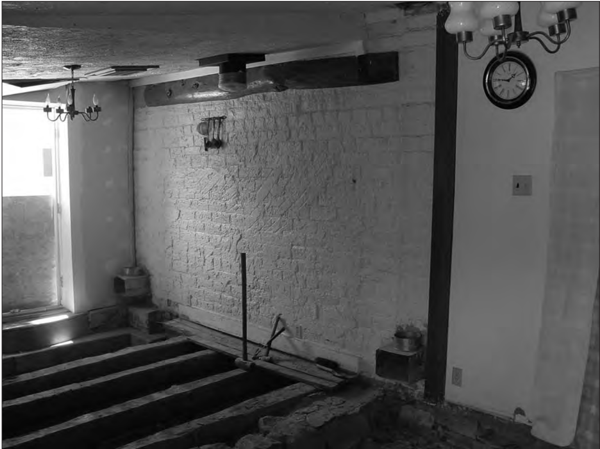
Figure 7. View of the central wall of the house in room block #3 from room block #4. Note the split log ceiling support bolted to the top of the wall, the walls bond pattern and adobe mud scratch coat can also be seen.
