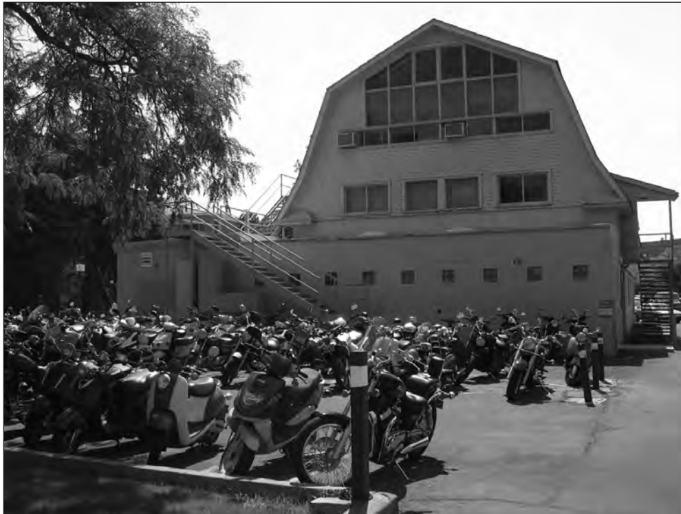
Figure 11. North side of the Barn, Summer 2009. Changes to the original diamond-shaped windows, additions for storage space, exterior fire escapes, and motorcycle parking detract from the classic lines of the 1919 Horse Barn. Photo courtesy, Mary Kay Gabriel, USU MOA.
