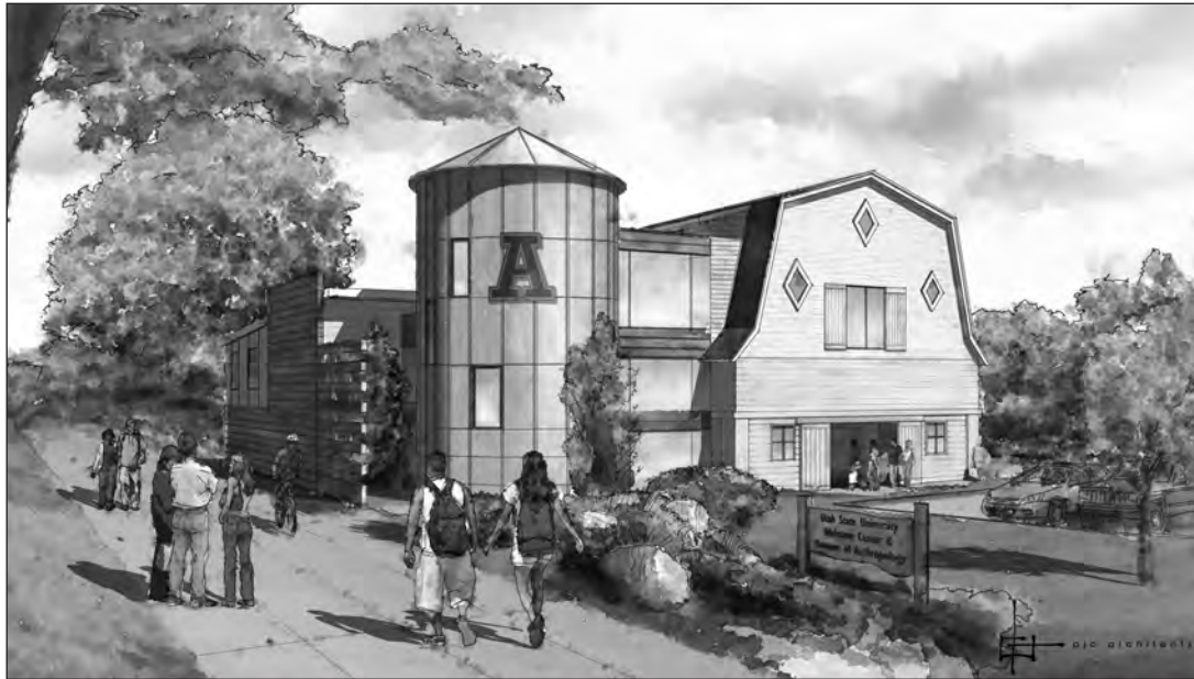
Figure 12. Conceptual view of the north side of the Aggie Barn and east-side additions. The silo houses an elevator and stairs; the addition behind the silo is a two-story learning center. Image courtesy, ajc architects, Salt Lake City.
