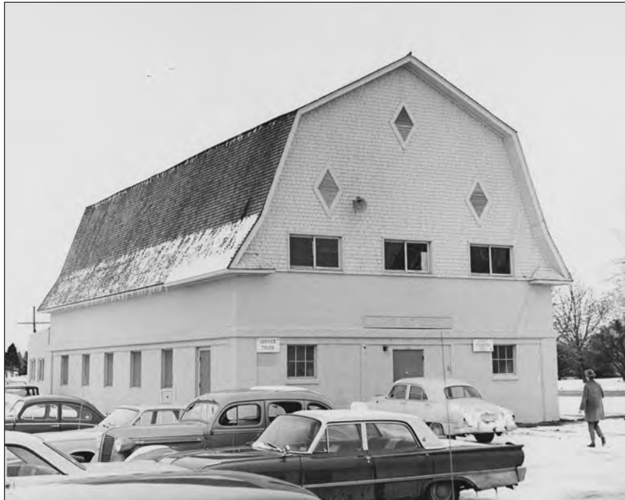
Figure 10. USU Art Barn, ca. 1962. Note that new square windows have been installed below the original diamond-shaped windows and the traditional sliding barn doors have been replaced with a standard door. Photo courtesy, USU Special Collections.
