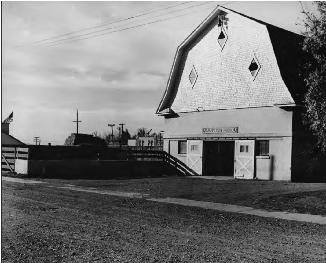
Figure 9. Horse Barn, ca. 1948). The features shown in this image of the Barn’s south face reflect the structure’s original (1919) appearance. Changes to the Barn’s windows and additions to the north and east sides post-date this photograph. Photo courtesy, USU Special Collections.
