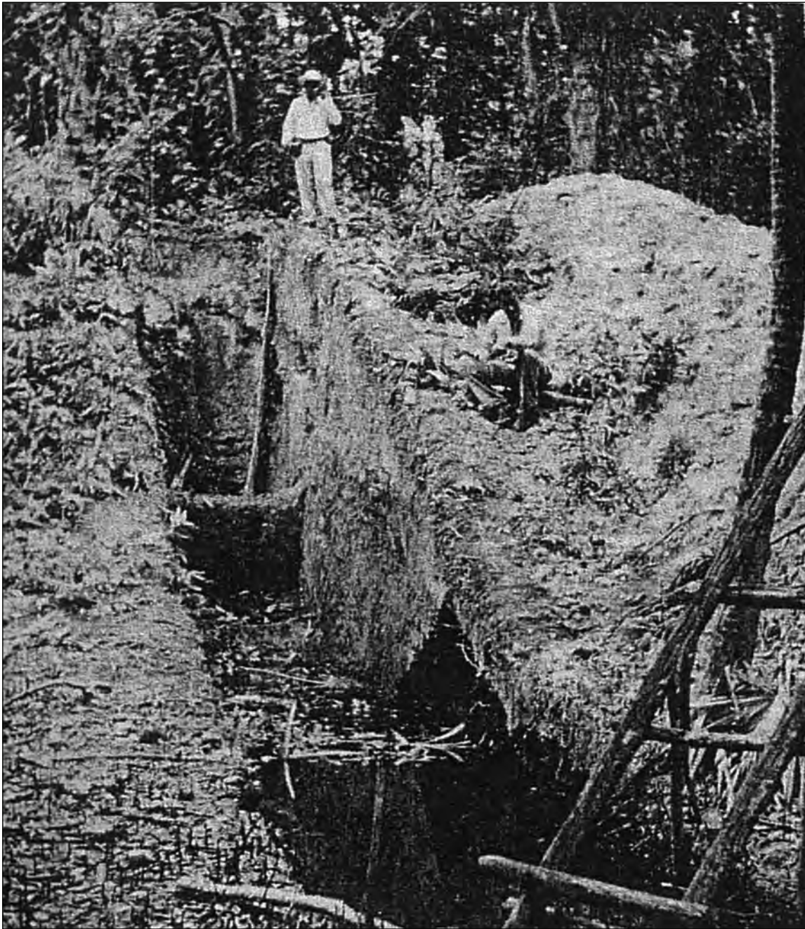
Figure 7. Excavations in Aguacatal in 1961.
