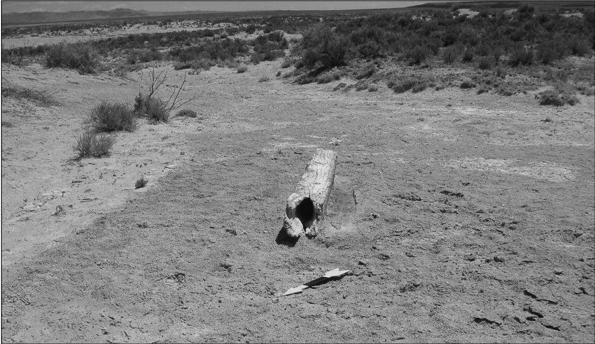
Figure 6. A section of bored-log pipe used in the construction of the Terrace Aqueduct associated with the Transcontinental Railroad.
