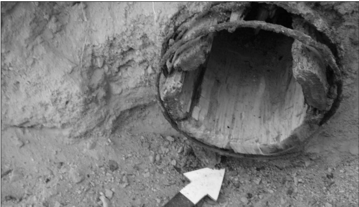
Figure 7. Section of wire-wound, wood-stave pipe used in the construction of the Rosebud Creek to Watercress Aqueduct associated with the Transcontinental Railroad.
