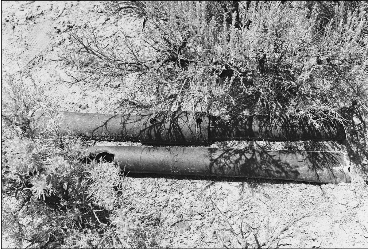
Figure 8. Longitudinally riveted sheet-metal pipe used in the construction of the Rosebud Creek to Watercress Aqueduct associated with the Transcontinental Railroad.
